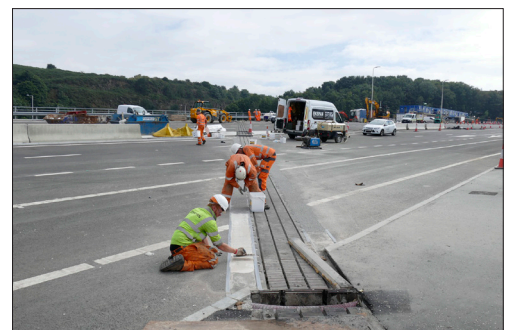
Expansion joint installation
