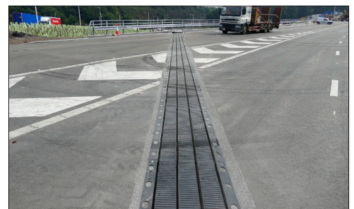
New installed TF900 expansion joint
