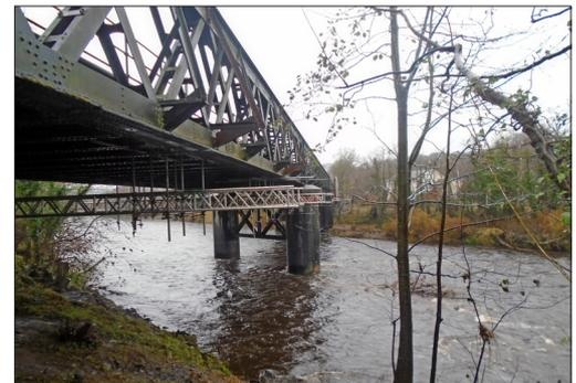
**Supplied:** USL Ekspan carried out an inspection of the 4 existing mechanical rocker bearings on the East and West abutments, followed by a subsequent inspection of the 4 no. pier bearings to ascertain their physical condition and their service capacity. All findings, conclusions and recommendations were provided in a report.
