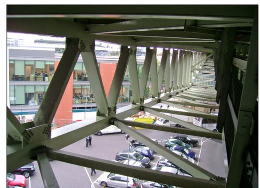
**Supplied:** USL Ekspan inspected eight (mechanical roller and spherical bearings) of the existing twelve bearings supporting the steel lattice girder section of the Boston Manor Viaduct. A report was compiled detailing their condition and serviceability.
