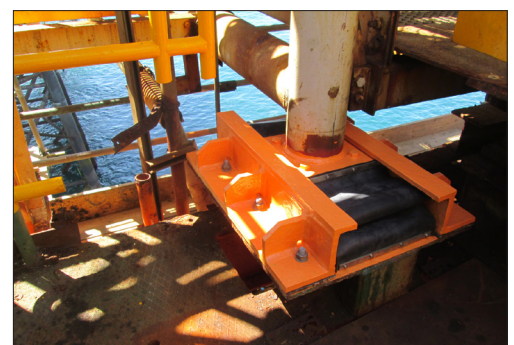
Bearing replaced complete with protective cover
